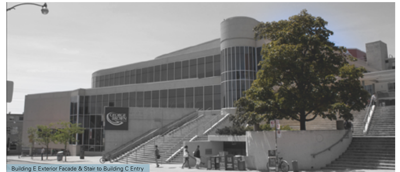
Building E Exterior Facade & Stair to Building C Entry
